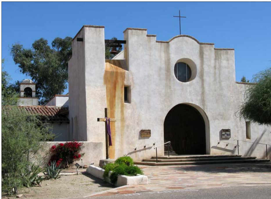
Saint Philip's in the Hills Episcopal Church was designed by famed Catalina Foothills architect Josias Joesler and built by developer John Murphey in 1936.
