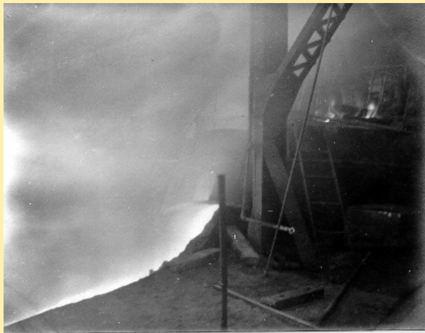
"Tapping" Furnace Settler, Washoe Smelter.
