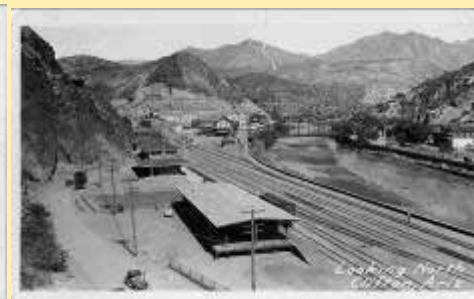
Looking North Clifton, Ariz.
