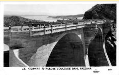
X3480 U.S. Highway 70 Across Coolidge
