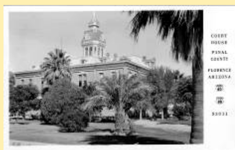
X3011 Court House Pinal County
