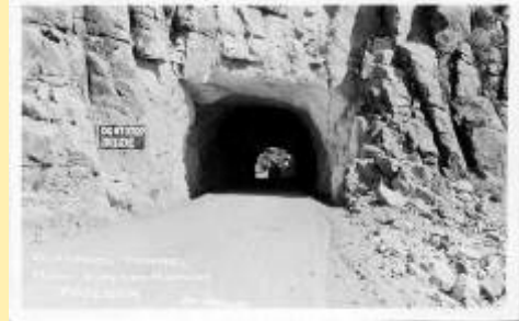
Claypool (4) Claypool Tunnel Miami-
