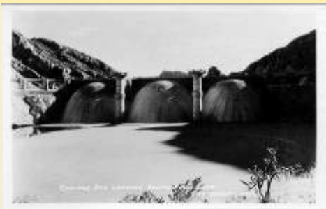
Coolidge (6) Coolidge Dam Looking
