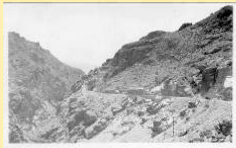
Picture (1) Road Near Claypool
