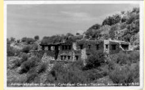
6-Y-438 Administration Building
