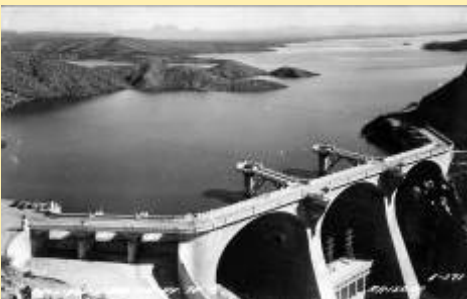
E-371 Coolidge Dam On Hy. 70 Arizona
