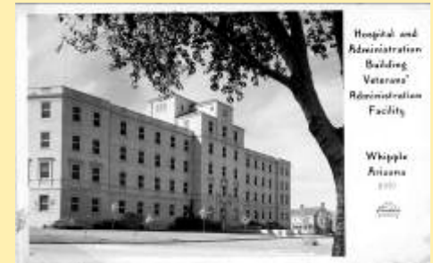
X530 Hospital and Administration Buildi
