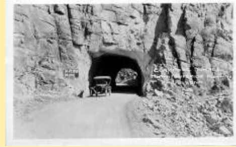
Claypool (6) Claypool Tunnel Miami-
