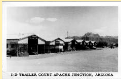
I-D Trailer Court Apache Junction, Arizona
