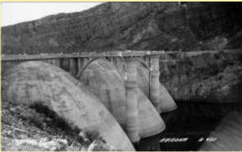
B-421 Coolidge Dam Arizona
