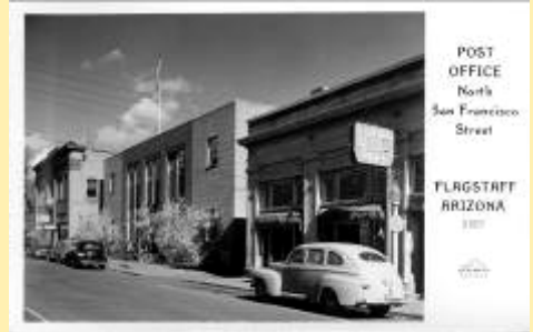
X607 Post Office North San Francisco Str
