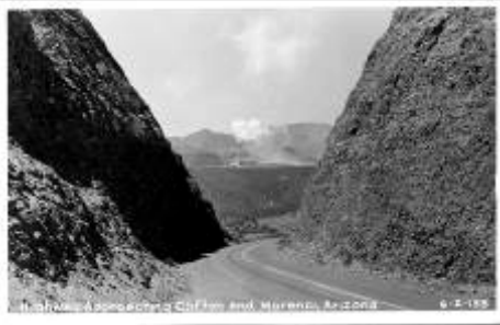
6-Z-135 Highway Approaching Clifton
