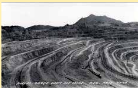
2-A-20, Phelps-Dodge Open Pit Mine,
