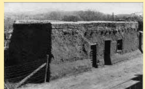
Picture 1, Adobe House
