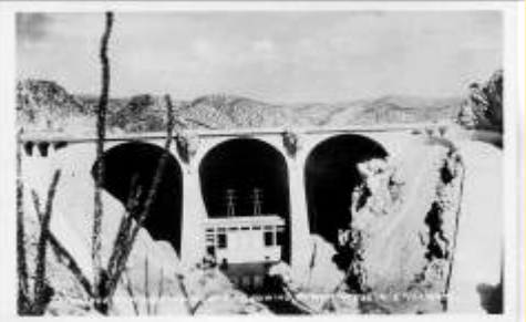
Coolidge (5) Coolidge Dam Looking
