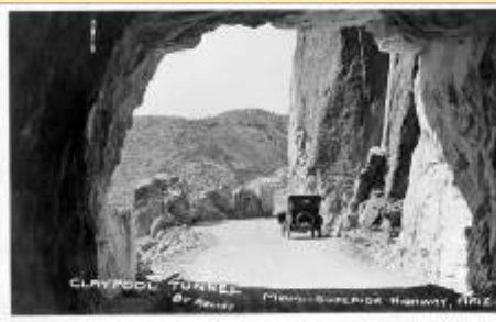
Claypool (5) Claypool Tunnel Miami-
