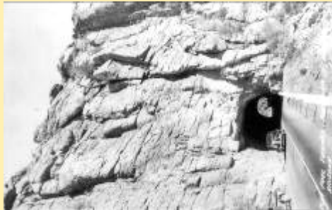
Clay Pool Tunnel, Superior Highway
