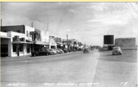
F-9 Main St. Casa Grande, Arizona
