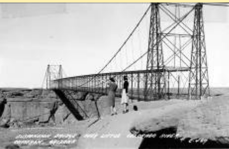
C-467 Suspension Bridge Over Little
