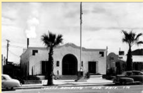
T 36, County Building-Ajo, Ariz.
