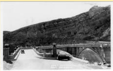
East Approach To Coolidge Dam, Arizon
