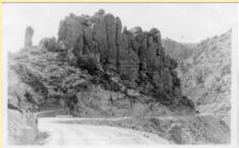
Picture (2) Road Near Claypool
