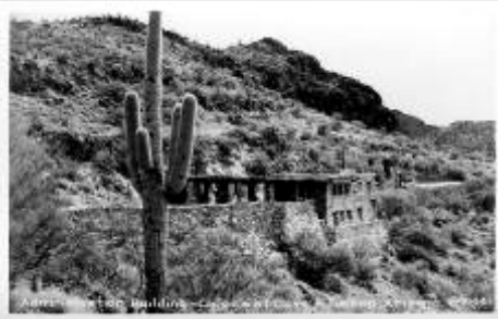
6-Y-441 Administration Building
