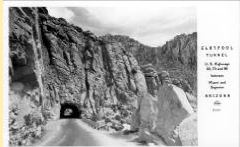
X3300 Claypool Tunnel
