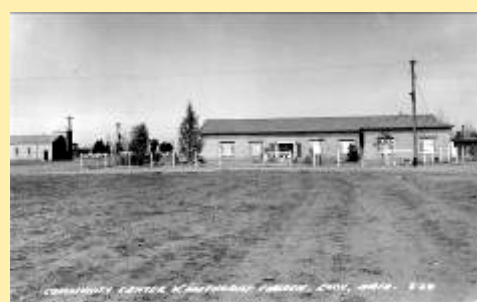
S-24 Community Center & Methodist Ch
