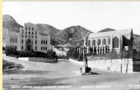
B 349, Court House And Catholic Church
