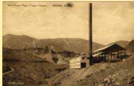
New Power Plant (Copper Queen) Bisbee, Ariz.
