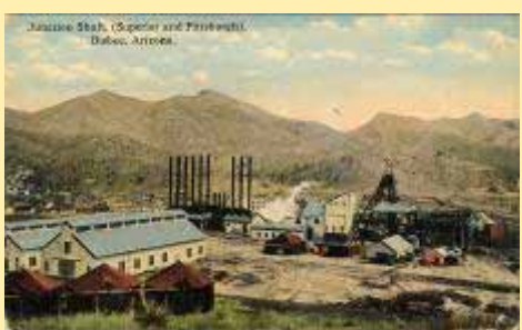
A-845 Junction Shaft, (Superior And Pittsb
