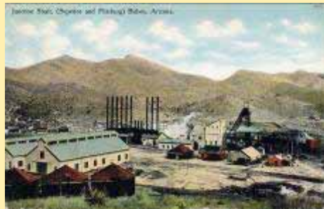
2075 Junction Shaft, (Superior and Pittsburg) Bisbee, Arizona
