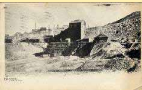
Bisbee, Arizona (20) Spray Shaft, Copper
