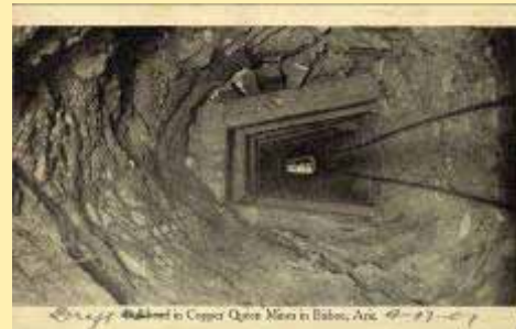
Bulkhead In Copper Queen Mines In Bisbee
