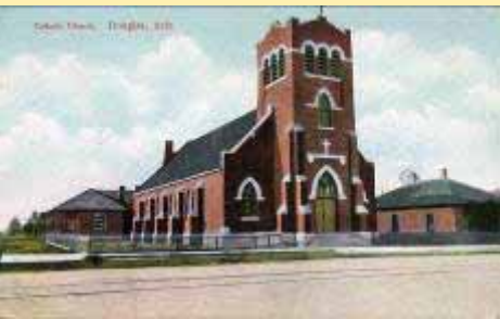
Catholic Church, Douglas, Ariz.
