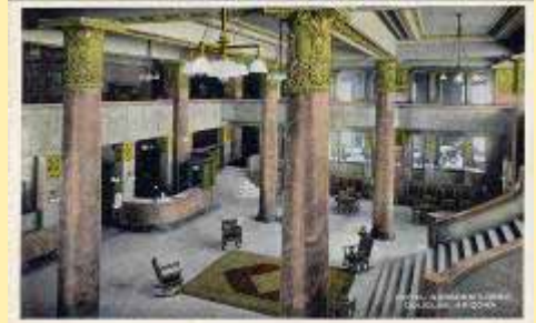
43966 (1) Hotel Gadsden Lobby, Douglas
