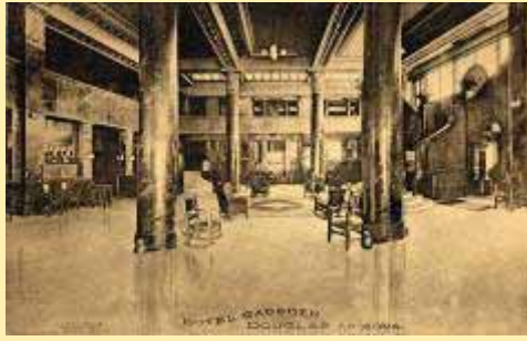
Hotel (4) Gadsden, Douglas, Arizona.
