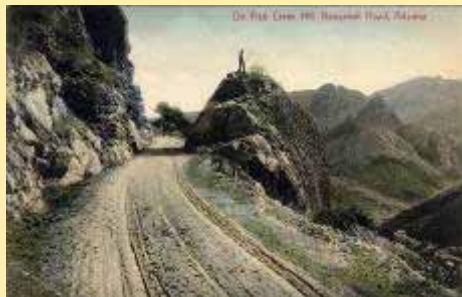
634 On Fish Creek Hill, Roosevelt Road
