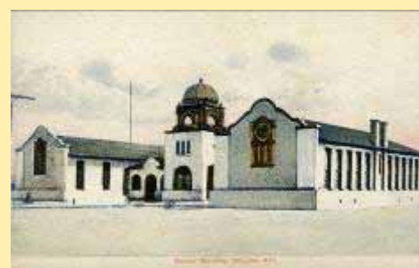
12604 C 8575 School Building, Douglas, A
