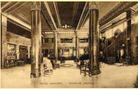
Hotel (3) Gadsden, Douglas, Arizona.
