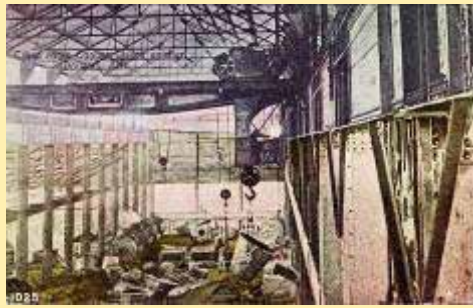
1025 Crane Room Copper Queen Smelter
