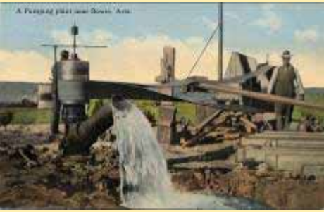
R-45940 A Pumping Plant Near Bowie, A
