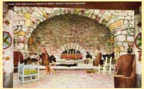
7506 The Fire Place, Hermit's Rest, Gran
