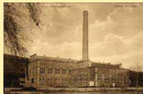
Power House, Miami, Arizona.
