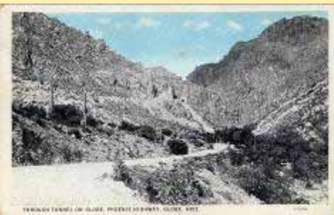
110194 Through Tunnel On Globe, Phoenix Highway, Globe, Ariz
