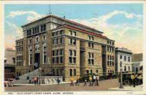
450 Gila County Court House, Globe, Ari
