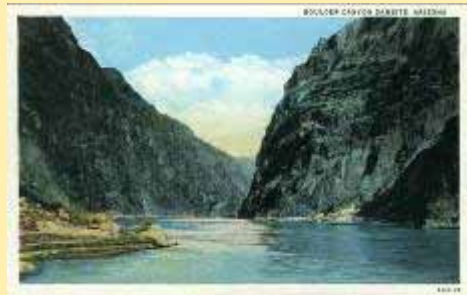
2455-29 Boulder Canyon Dam site, Arizon
