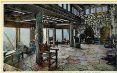
H-1343 View, Hermit Rest, Windows Ov
