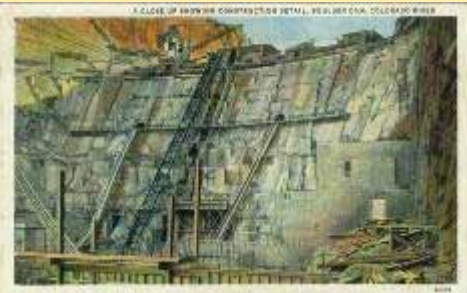
4A309 A Close-Up Showing Construction
