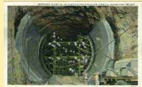
2A1183 Entrance To One Of the Four 56
