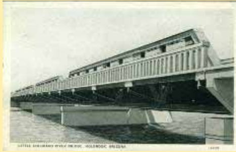
122500 Little Colorado River Bridge, H
