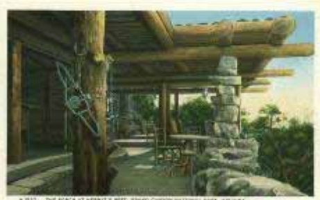
H-1537 A-98048 The Porch At Hermit's
