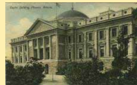
21542 Capitol Building, Phoenix, Arizona
