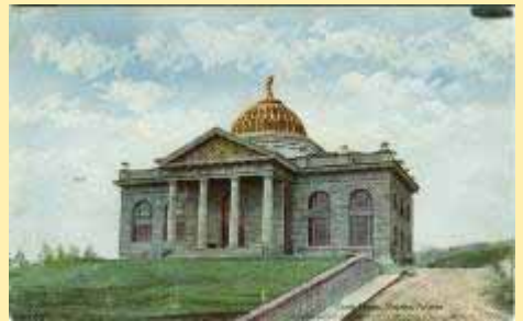
2702 Court House, Nogales, Arizona.
