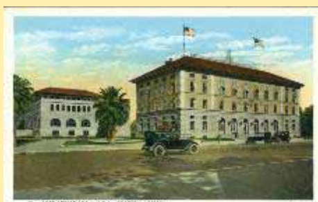
121. 112047 Post Office And Y.M.C.A.,
