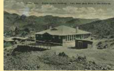
Oatman, (4) Ariz. Public School Building.
