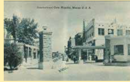
D 1708 International Gate, Nogales, Mexico
