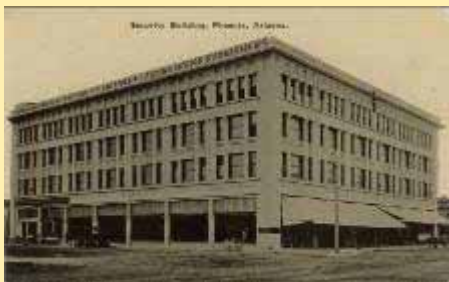
209. Security Building, Phoenix, Arizona.
