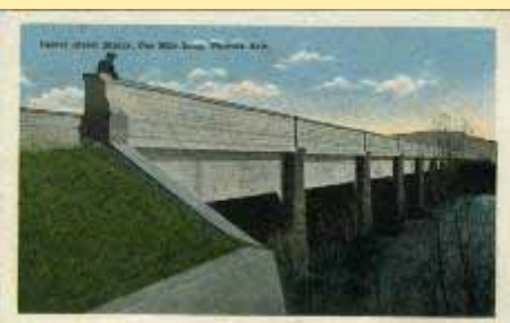
15853 Center Street Bridge, One Mile Lo
