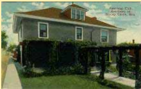
38758 American Club, Residence Of Brac
