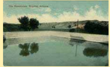
38722 The Natatorium, Nogales, Arizona
