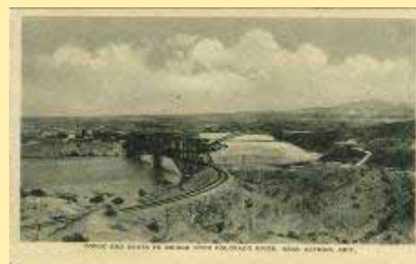
Topoc And Santa Fe Bridge Over Colorad
