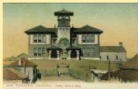
5829 Nogales, Arizona. Public School B
