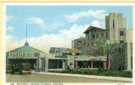
246 4638-29 Entrance, Arizona Biltmore,
