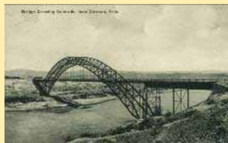
Bridge Crossing Colorado, Near Oatman,
