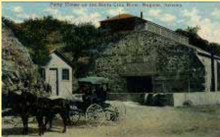
38746 Pump House On The Santa Cruz Riv
