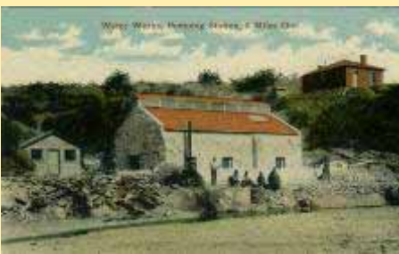
38730 Water Works, Pumping Station, 8
