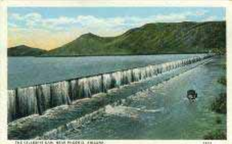
104930 The Gillespi Dam, Near Phoenix,
