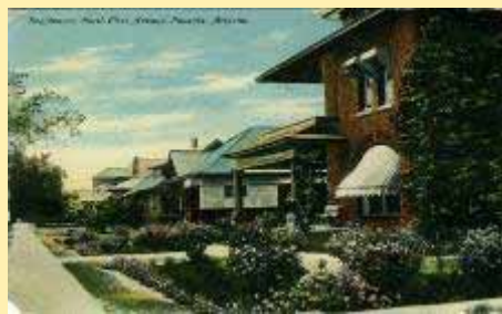
A-9143 2593 Residence, North First Ave
