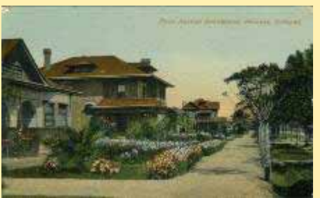
9869 First Avenue Residences, Phoenix,
