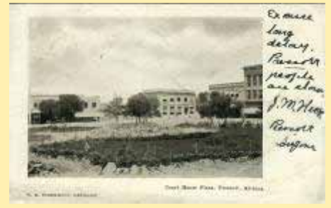
Court (2) House Plaza, Prescott, Arizona.
