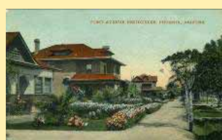
9869 First Avenue Residences, Phoenix,
