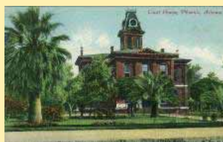
A R 23 Court House, Phoenix, Arizona
