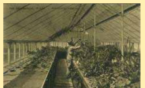
The Greenhouse, Plaza, Prescott, Arizona
