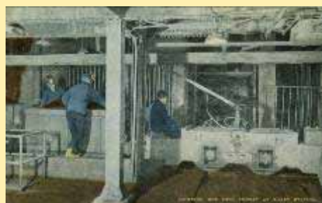
30376 Dumping Ore Into Pocket At Shaft
