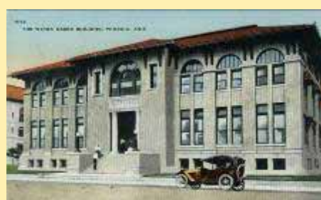
4114 The Water Users Building, Phoenix,
