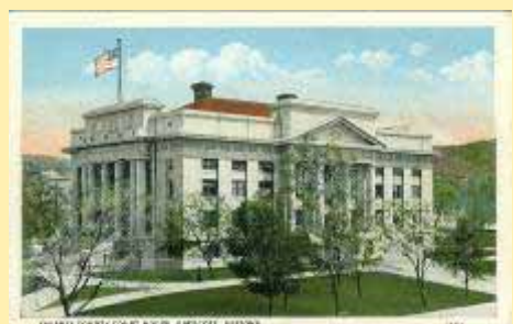
104455 Yavapai County Court House, Pr
