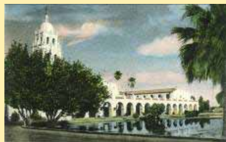
Looking (4) South-East On Grounds St. Fr
