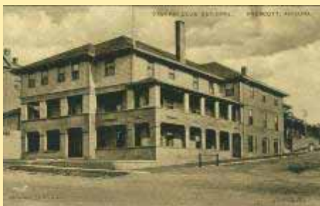
Yavapai (3) Club Building. Prescott, Ariz.
