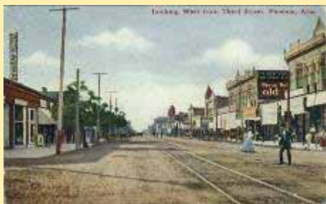
Looking (1) West From Third Street, Pho
