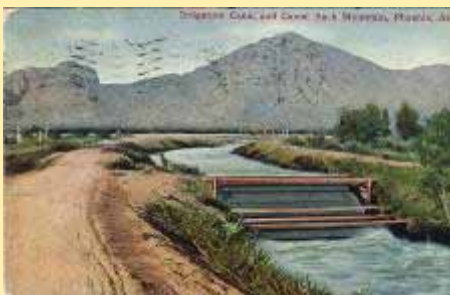
Irrigation (1) Canal And Camel Back Mo
