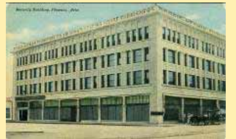
A-12554 2880 Security Building, Phoenix
