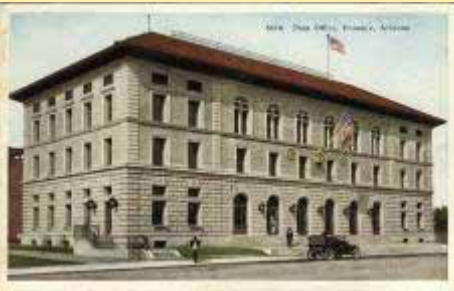
5410. Post Office, Phoenix, Arizona
