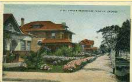
9869 First Avenue Residences, Phoenix,
