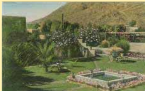
Patio (2) Of Main Building Jokake Inn Jo
