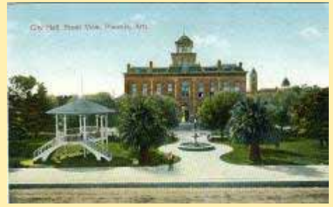
5236. City Hall, Front View, Phoenix, Ar
