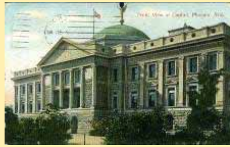
5235. Front View Of Capitol, Phoenix, A
