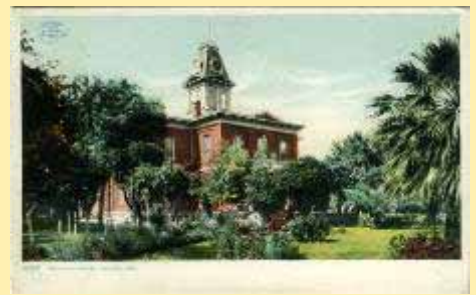
6306 The Court House Phoenix, Ariz.
