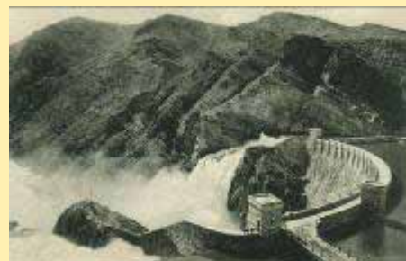
Roosevelt (11) Dam, Arizona.
