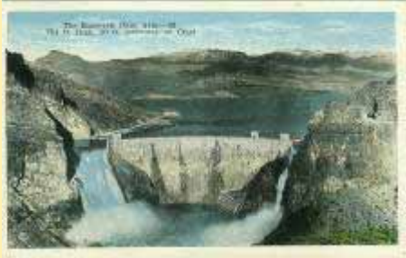
33 25468 The Roosevelt Dam, Ariz.
