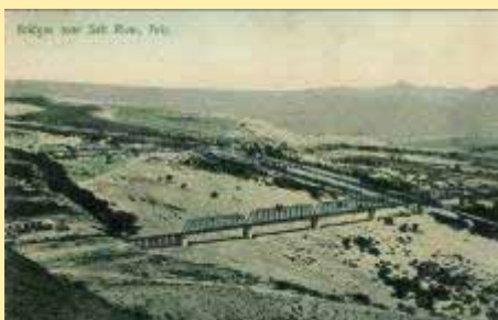
20245 Bridges Over Salt River, Ariz.
