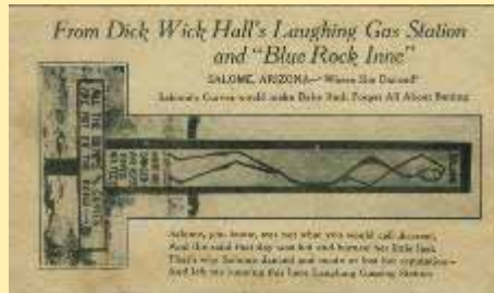
From Dick Wick Hall's Laughing Gas Station
