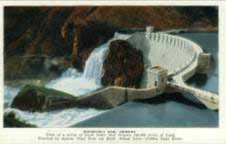
10524-N Roosevelt Dam, Arizona
