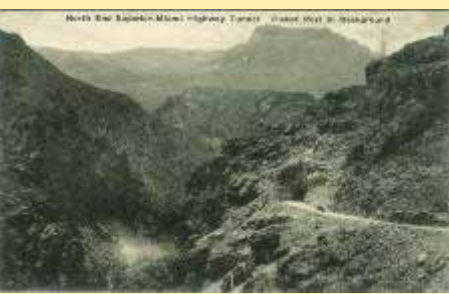
North End Superior-Miami Highway Tun
