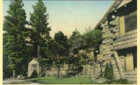
Main (2) Building Jokake Ranch Springerville,
