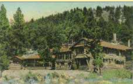
Main (3) Building Jokake Ranch Springerville,
