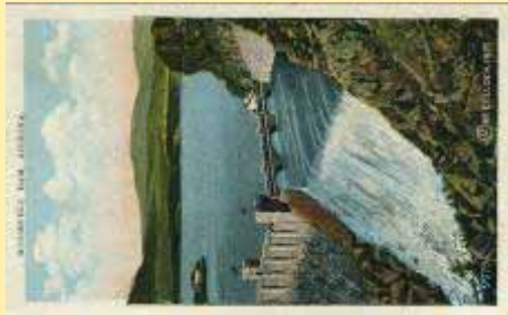
9775 Roosevelt Dam, Arizona.
