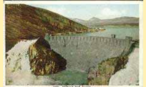
16003 Roosevelt Dam, Arizona
