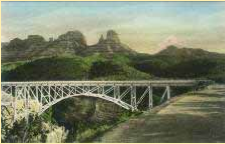
Wilson Canyon Bridge Near Oak Creek C
