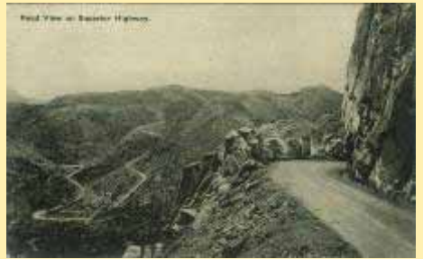
Road (1) View On Superior Highway.
