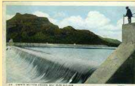
216. Granite Reef Dam Arizona, Salt River
