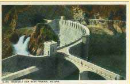
H-2395 55057 Roosevelt Dam Near Phoe
