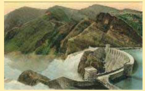
The (7) Roosevelt Dam, On Apache Trail
