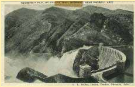
Roosevelt (16) Dam, On Apache Trail Hi
