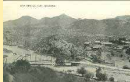
New Bridge, Ray, Arizona
