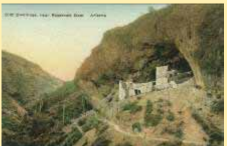
Cliff (3) Dwelling, Near Roosevelt Dam
