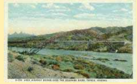
H-2799 Arch Highway Bridge Over The
