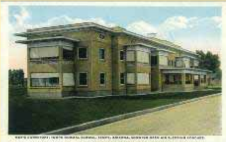
R-81743 Men's Dormitory, Tempe Norm
