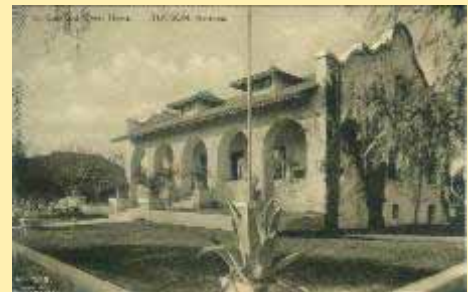
208 An East 3rd Street Home. Tucson, Ar
