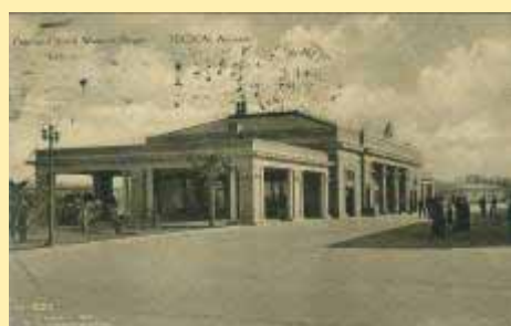
232 Paso And South Western Depot, Tucs
