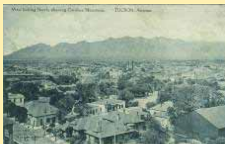
152 View Looking North, Showing Catal
