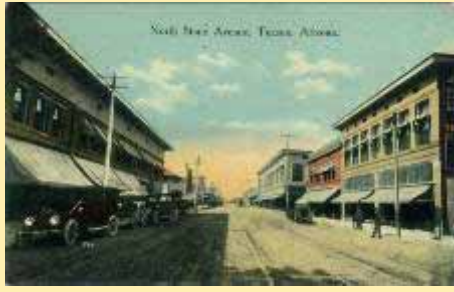
T. A. 228 North stone Avenue, Tucson, Ar
