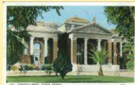
263 26985 Carnegie Library, Tucson, Ari
