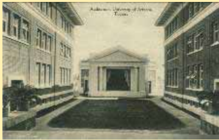
Auditorium, University Of Arizona, Tucs
