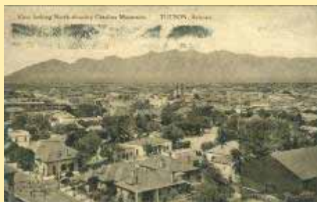
203 View Looking North Showing Catalina
