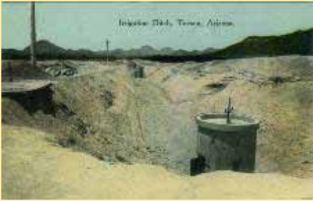
T. A. 231 Irrigation Ditch, Tucson, Arizona
