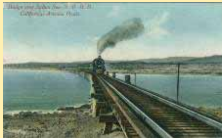
AR 28 Bridge Over Salton Sea—S.P.R.R.
