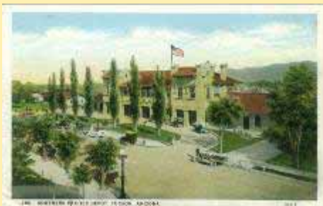
260 87312 Southern Pacific Depot, Tucso
