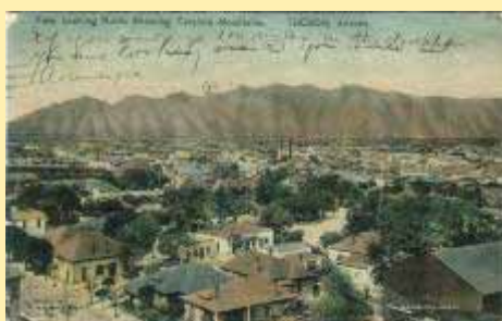
View Looking North Showing Catalina M
