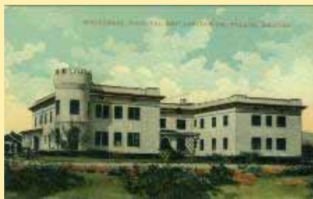
9850 Whitewell Hospital And Sanitarium, Tucson, Arizona
