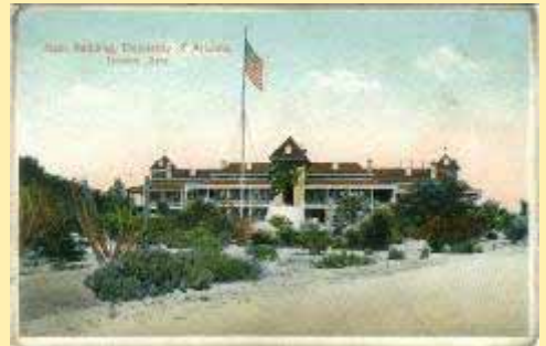
5190 Main Building, University Of Arizo
