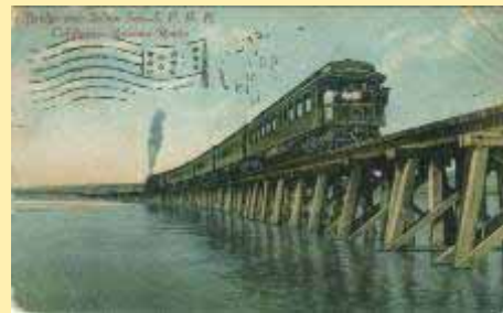
AR 29 Bridge Over Salton Sea-S.P.R.R.
