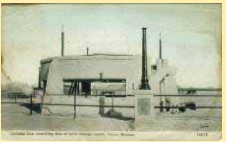
16210 Cylinder Gate Controlling Flow Of
