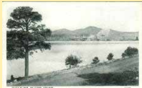
110857 Santa Fe Dam, Williams, Arizona
