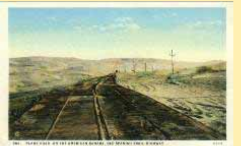
508. 103675 Plank Road, On The Americ
