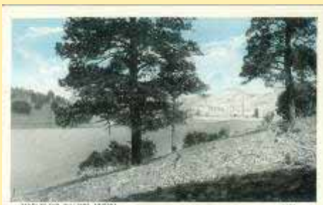
110830 Santa Fe Dam, Williams, Arizona
