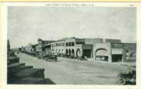
5907 Main Street Looking North, Yuma,
