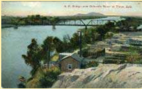
AR17 S. P. Bridge Over Colorado River
