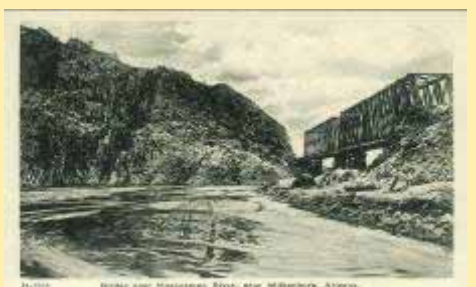
H-2974 Bridge Over Hassayampa River, N
