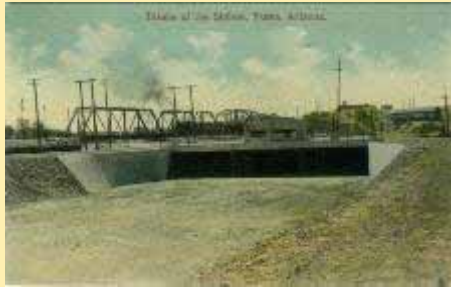
22644 Intake Of The Siphon, Yuma, Ariz
