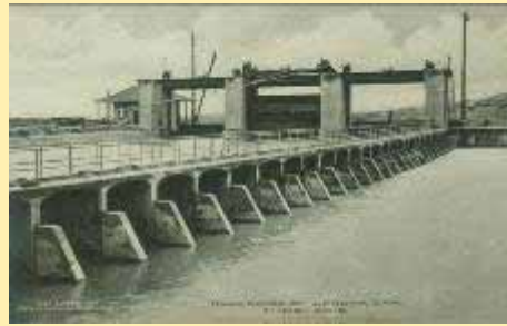
Head Gates At Laguna Dam, Yuma, Ariz.
