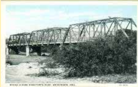
BS-110179 Bridge Across Hassayampa R
