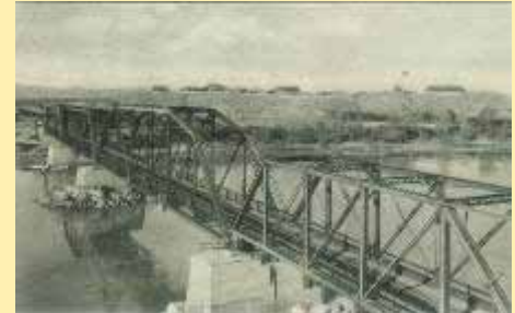
Southern (2) Pacific Railway Bridge. Yum
