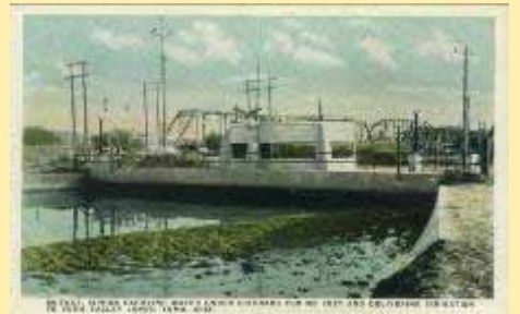
56845 In-Take Siphon Carrying Water Un
