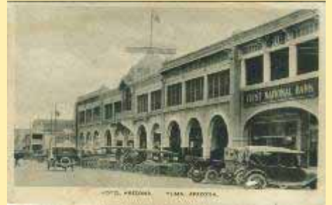
Hotel Arizona. Yuma, Arizona.
