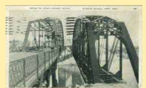
5911 Highway Bridge, Yuma, Ariz.
