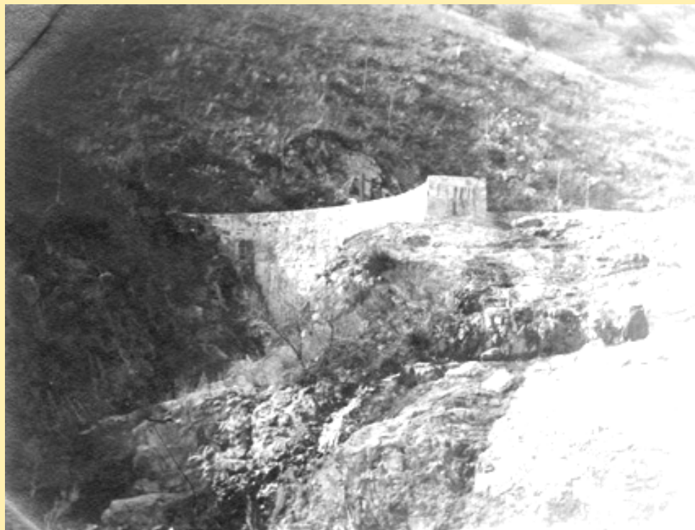
Dam Below "El Oro"
