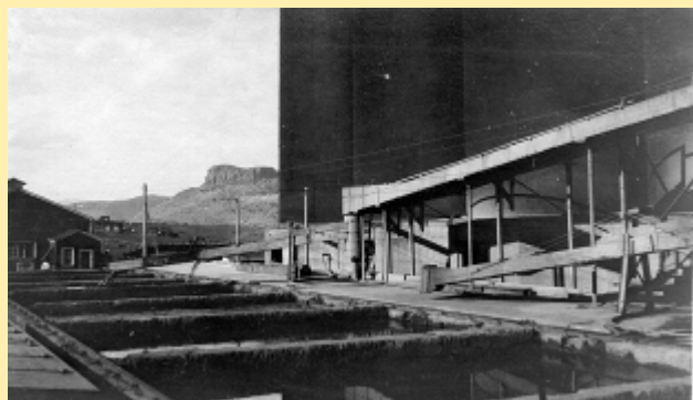
Main Concentrate Tanks – Distributing Arm Launderers on arcs. Traveling Crane and bucket loads out of bins into cars.
