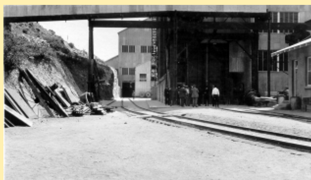
Inspiration Copper Co. Shaft Entrance.
