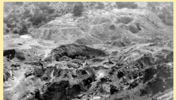
Mexicans working over caved surface of Old Dominion fault about 200 ft. below crest of hanging wall.
