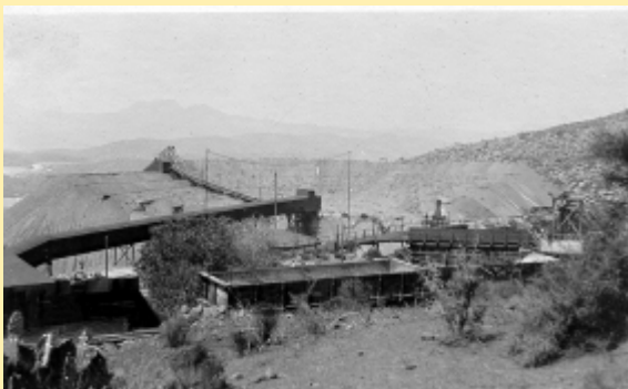
Old Dominion Tailings Disposal. Radial launder on tracks.
