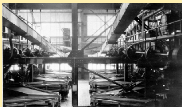
Inspiration Mill, Double Deck Deister Tables and Drag Classifiers.
