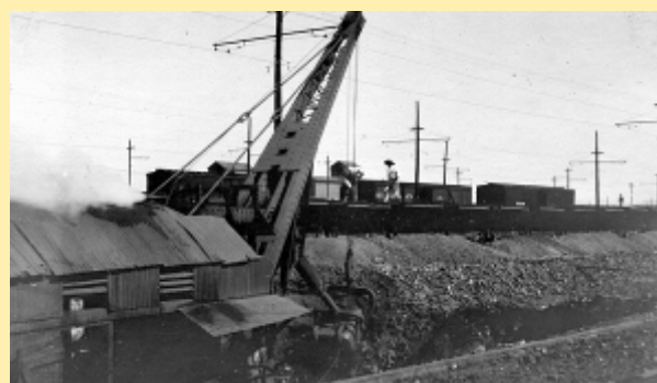
Two Views of Copper Queen Bedding Troughs Layers of ore, lime molten slag, etc. dumped in and spread with machine in left picture. Reclaiming done with bucket hoist in right picture.
