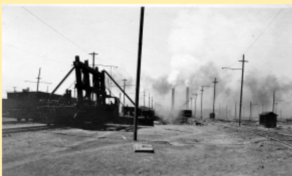
Two Views of Copper Queen Bedding Troughs Layers of ore, lime molten slag, etc. dumped in and spread with machine in left picture. Reclaiming done with bucket hoist in right picture.
