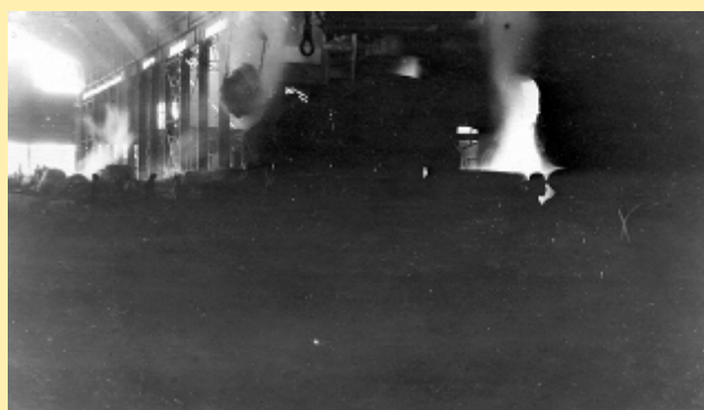
Copper Queen Smelter Converters blowing.
