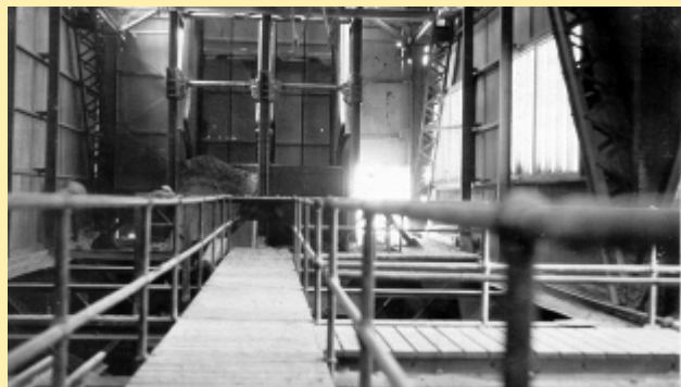
Inspiration Copper Co., Skip Dumps
