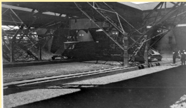
Two Views of Calumet & Arizona Smelter – Douglas, Ariz. Ore Bedding – Ore is distributed by belt conveyers (also fluxes). Machine shown takes lateral slices, scraping on to belt conveyor in side ditch.
