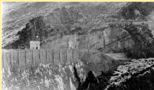
Globe to Phoenix – Roosevelt Dam – East End – Main Road above.
