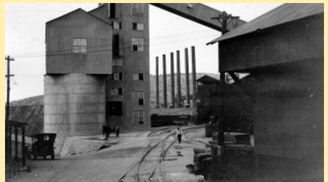
Storage bin at Old Dominion Shaft, Globe, Arizona.
