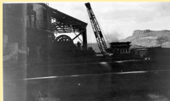
Oliver Filters and Concrete Concentrate Tanks. Clam shell bucket crane loading box cars through traveling hopper.
