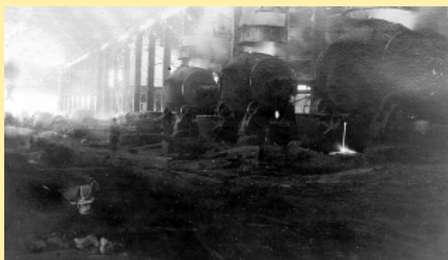
Copper Queen Smelter Converters blowing.
