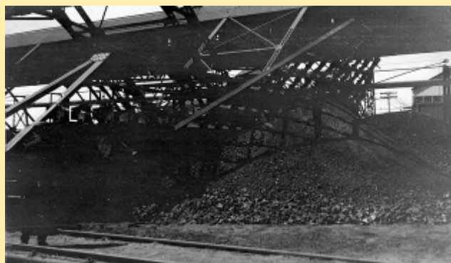
Two Views of Calumet & Arizona Smelter – Douglas, Ariz. Ore Bedding – Ore is distributed by belt conveyers (also fluxes). Machine shown takes lateral slices, scraping on to belt conveyor in side ditch.
