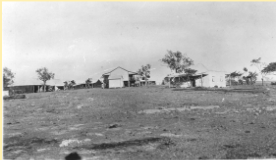
General View Lawn Hill Station Buildings.
