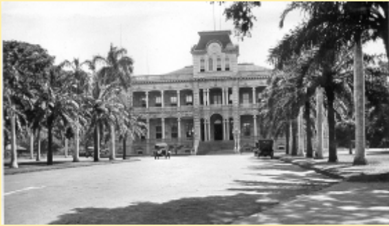
Capital Building – Honolulu.
