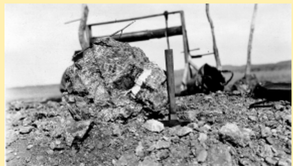
Specimen – Watsons Lode, Sphalerite cemented breccia from 100' crosscut.
