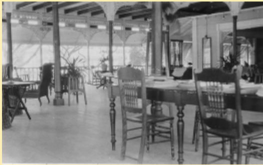
Verandah – Park Hotel – Georgetown – B.G.
