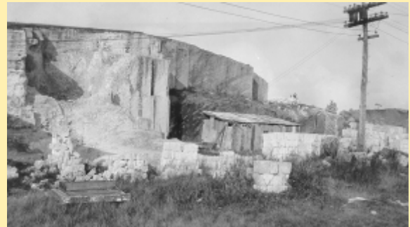
Bermuda – Quarry for Coral Rock building Blocks.
