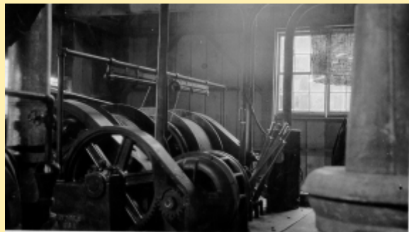
Minnie Moore Mine, Hoist & Compressor, March 1924.
