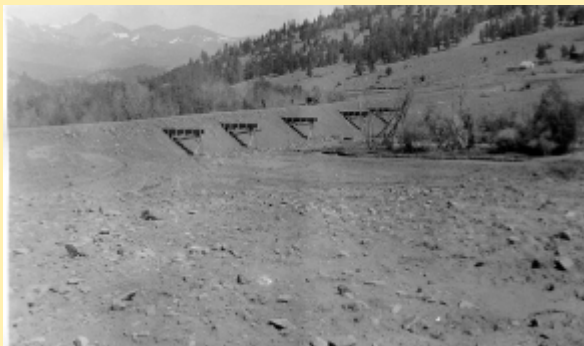
Building Dam #5, Rawley 1927.
