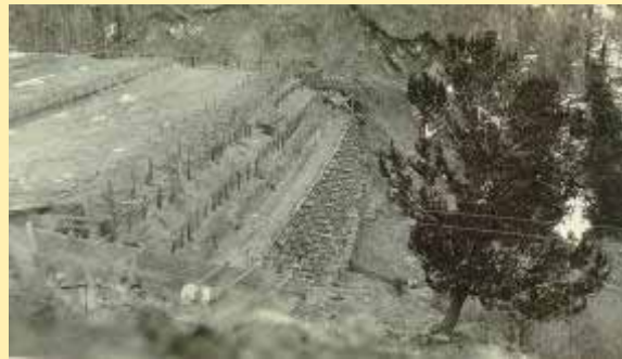
Rawley – 1928 Mill Dam – Operating.
