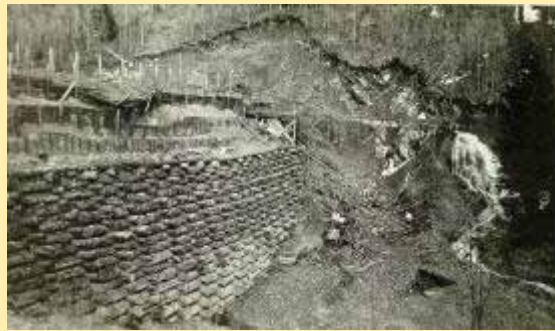
Rawley – Mill Dam 1928 Operating.
