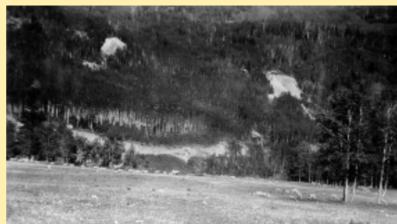
Tunnels on Newman Hill – Rico – Colorado 1924.
