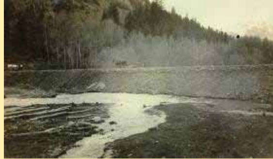
Outlet – Dam #3, Rawley 1928 High Water.
