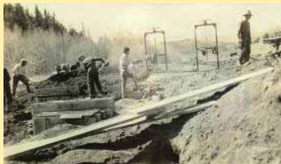
Setting pipes in Dam #3 – Rawley, 1928.
