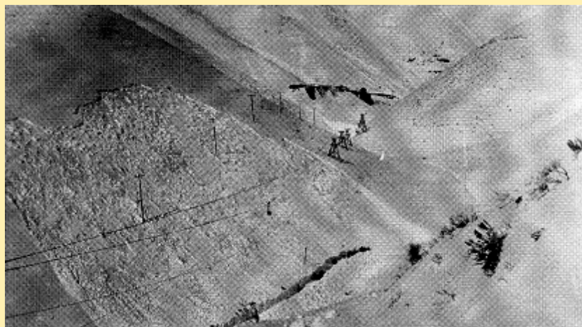
Up North Star Gulch, Shoveling road through snow slide.
