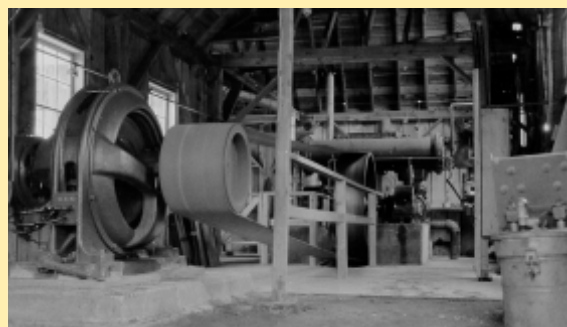
Minnie Moore Mine, Hoist & Compressor, March 1924.
