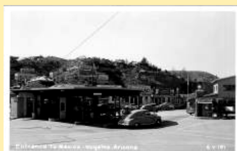
6-Y-151 Entrance To Mexico-Nogales A
