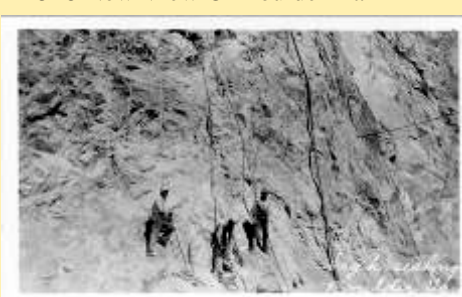
High Scaling Boulder Dam
