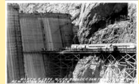
388 March 9, 1934 When Boulder Dam
