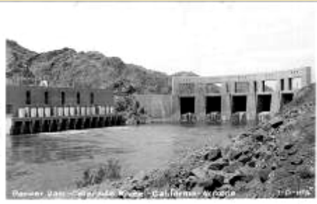
7-D-154 Parker Dam—Colorado River-C
