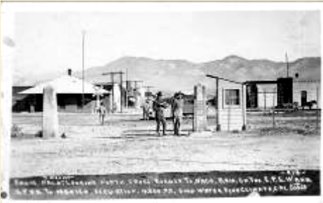
214 From, Naco-Looking North Cross Bo
