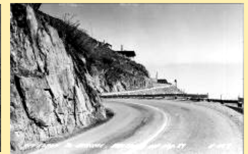
E-157 Approach To Jerome, Arizona On
