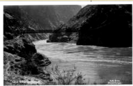
Kaibab Bridge Over Colorado
