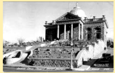
C-84 Santa Cruz County Court House
