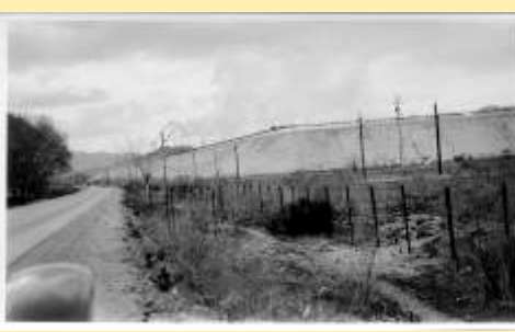
Picture (1) Smelter Of Copper Mine
