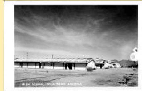
High School-Gila Bend, Arizona
