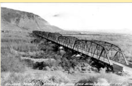
C-37 Gillespie Bridge Highway 80 Near Gi
