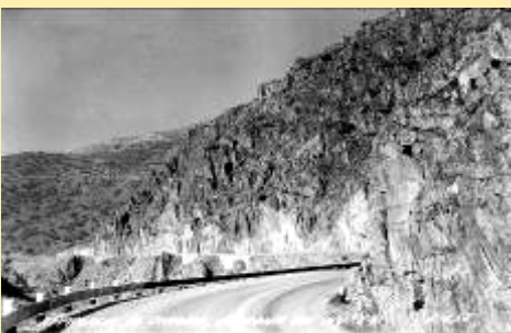
E-158 Approach To Jerome, Arizona On
