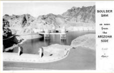
F1827 Boulder Dam As Seen From The A
