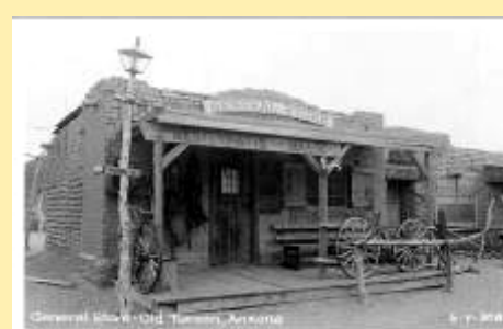
6-Y-308 General Store-Old Tucson, Arizo
