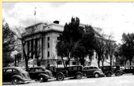
C-296 Court House Prescott, Arizona
