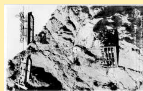
Going On Shift In Cable With Skip-Hoov
