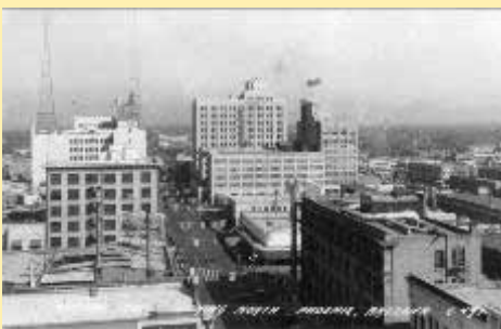
C-491 Central Ave, Looking North Phoeni
