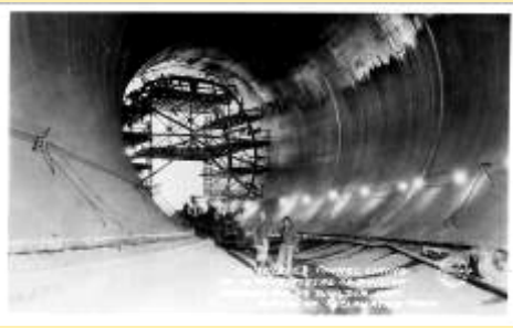
Completed Tunnel Lining At Intake Port
