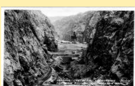
Looking Upstream Excavation For Dam F
