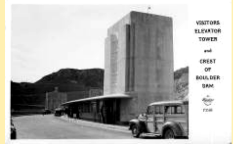
F3586 Visitors Elevator Tower and Crest
