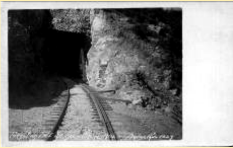
1027 Tunnel On P & E Near Poland, Ariz.
