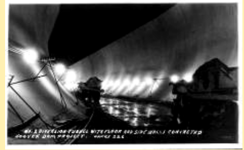
226 No. 2 Diversion Tunnel With Floor
