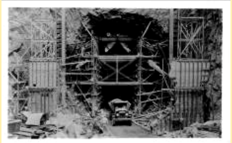
Picture (6) Dam Being Built Truck In Fro
