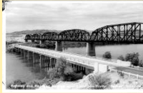
7-D-152 Highway And Railroad Bridge
