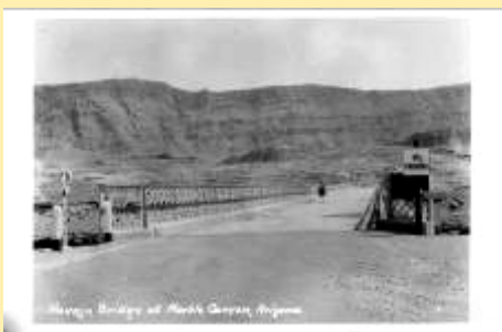
Navajo Bridge At Marble Canyon, Arizona
