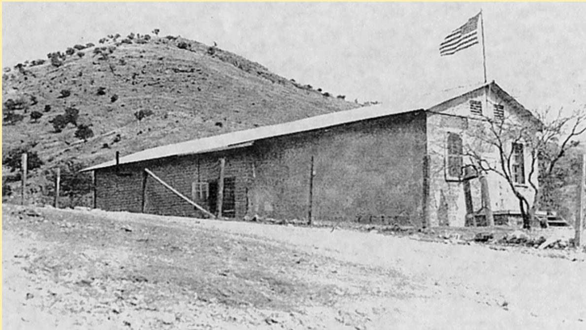
This Ruby school was expanded to accommodate eight grades and as many as 150 students. (Tallia Pfrimmer Cahoon private collection)
