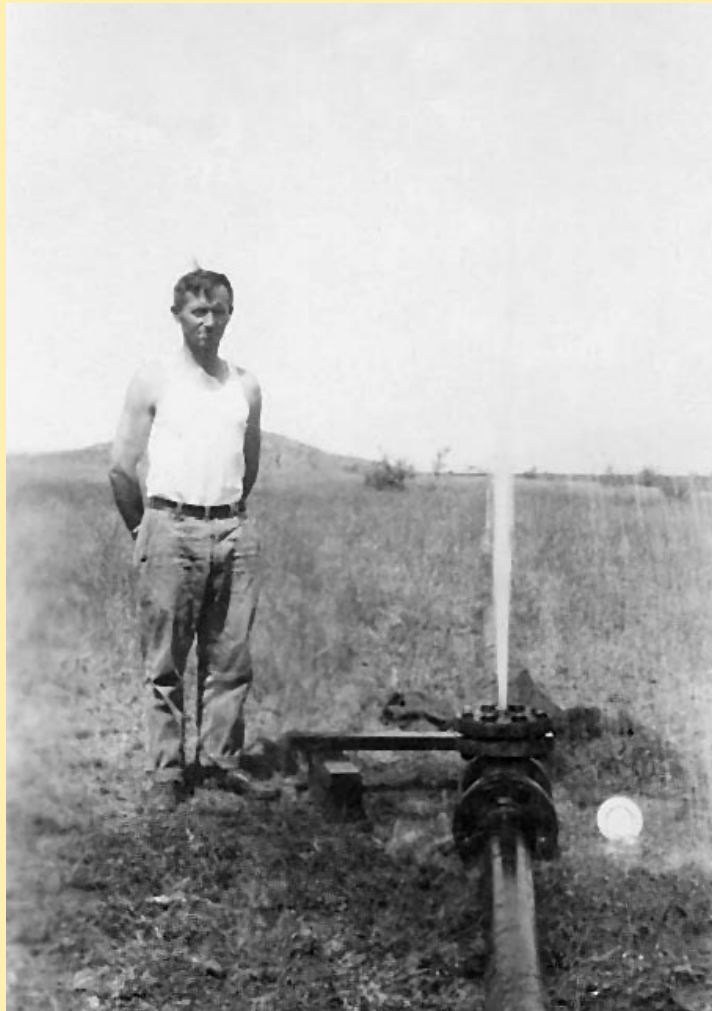
My dad, Walter Pfrimmer, standing next to a connection joint on the new water pipeline. (Tallia Pfrimmer Cahoon private collection, 1929)
