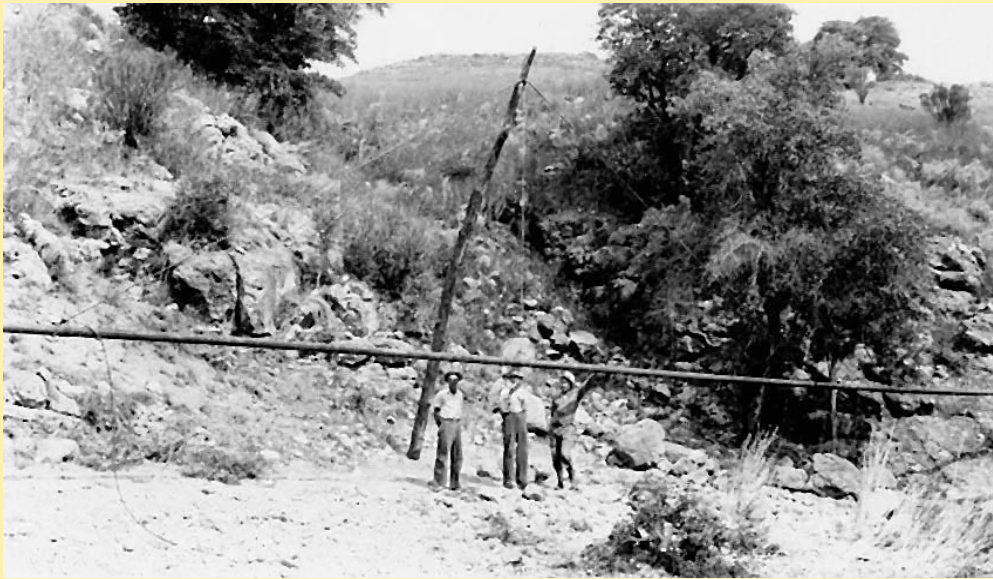
The 17-mile long, 4-inch pipeline was completed in 1930. (Tallia Pfrimmer Cahoon private collection)
