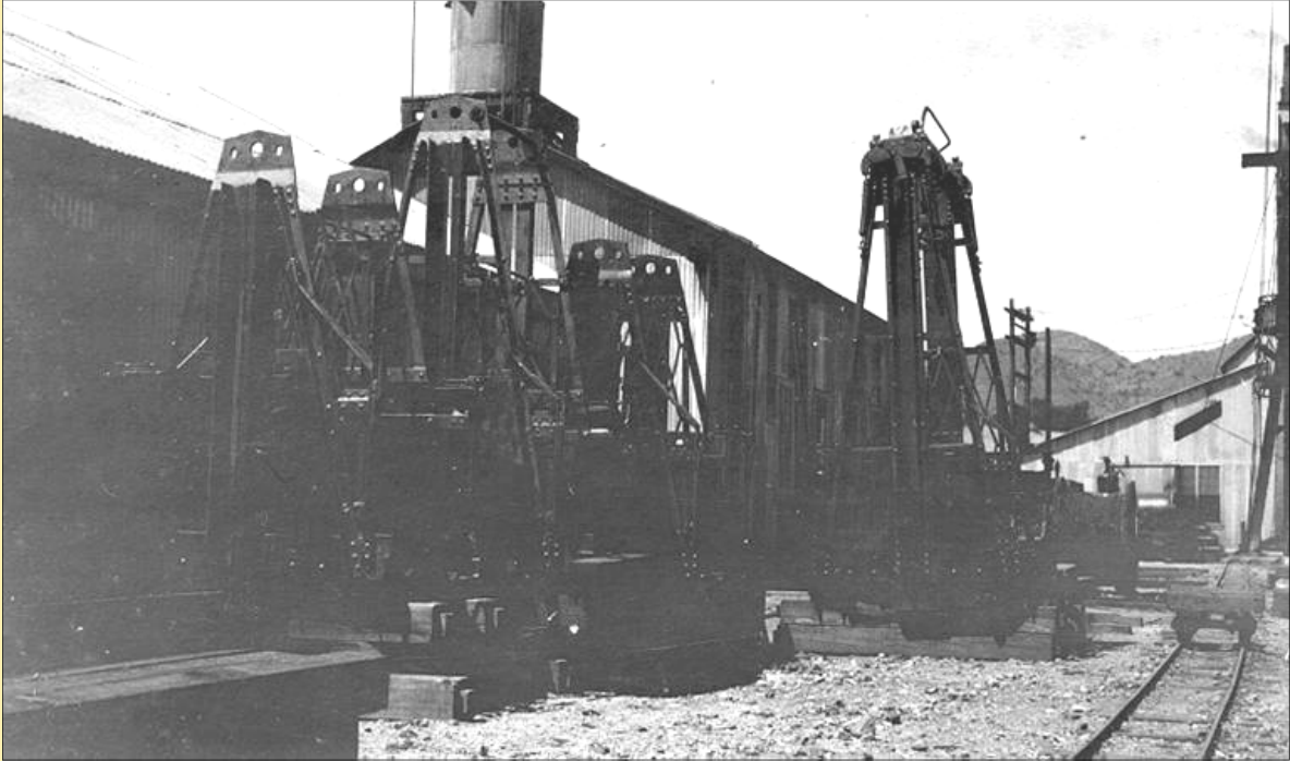
These cages at the Junction Shaft were used to lower groups of miners to the working levels below ground. (Photo by Ambrose E. Ring, 1916)
