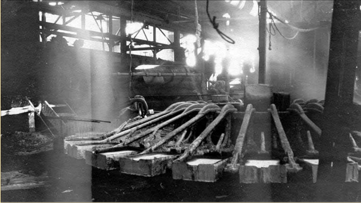
This spider-like apparatus is the casting machine at the Copper Queen smelter. (Photo by Ambrose E. Ring, 1916)
