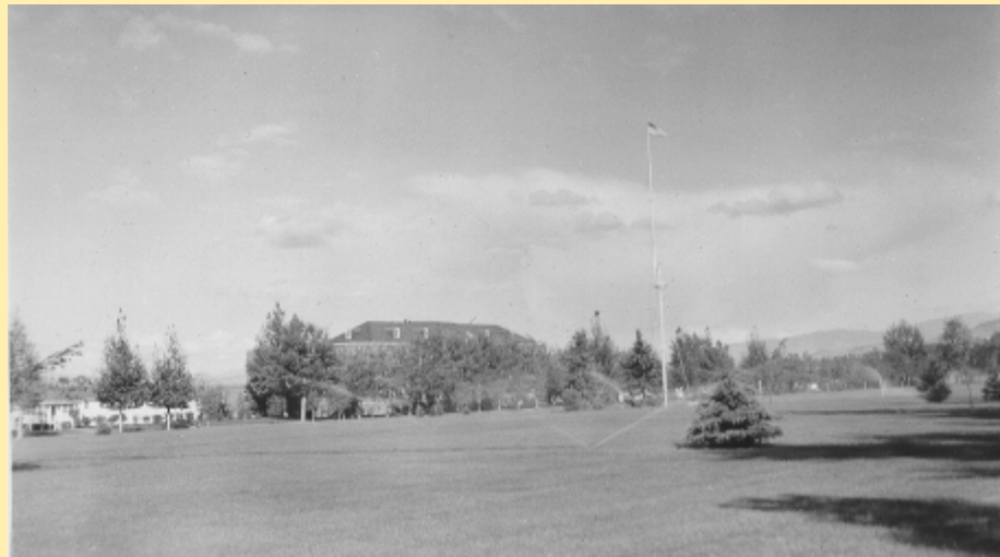
Ft. Harrison – Mont. – June 1951, Main Hospital building.
