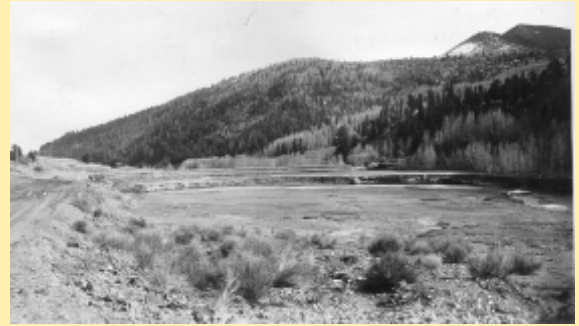
Rawley – 1930 – Old #3 Dam.
