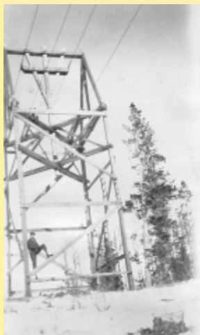
Tower on Tram.
