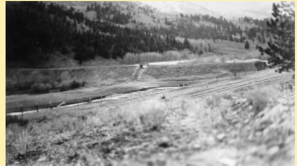
Rawley – 1930 – Old #4 Dam.
