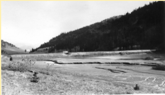
Rawley – 1930 Old #4 Dam.
