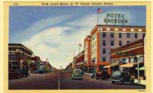
C-2 South Toward Mexico, On "G" Ave
