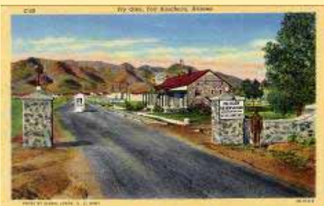
C-29 Fry Gate, Fort Huachuca, Arizona
