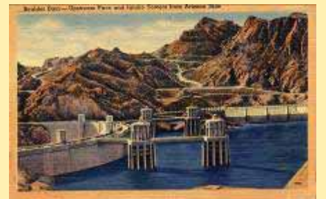
74662 Boulder Dam-Upstream Face And
