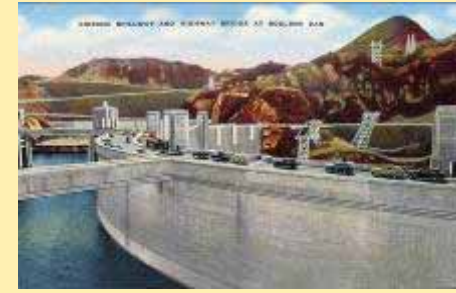
28107N Arizona Spillway And Highway
