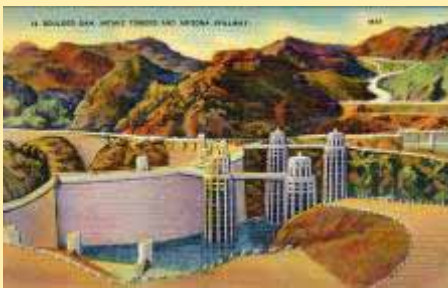
14 Boulder Dam, Intake Towers And Ari
