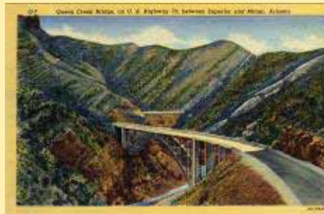
G-7 Queen Creek Bridge, On U. S. Highw
