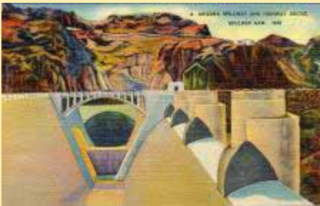
4 1651 Arizona Spillway And Highway
