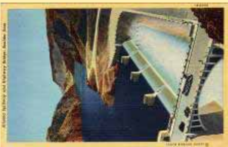
1B-H2430 Arizona Spillway And Highwa
