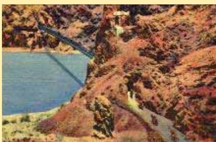
G.C.-6 Foot Of Kaibab Trail And Bridge
