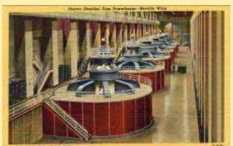
1B-H408 Hoover (Boulder) Dam Power
