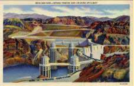
6A-H2036 Boulder Dam-Intake Towers A
