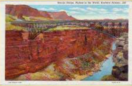
229 2505-29-N Navajo Bridge, Highest I
