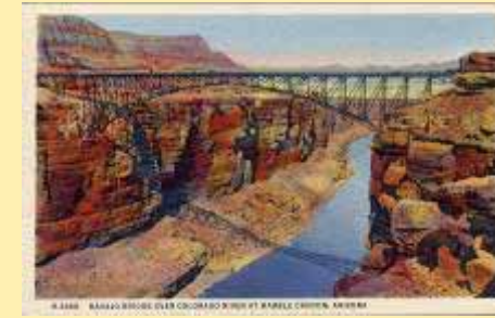
H-3960 Navajo Bridge Over Colorado
