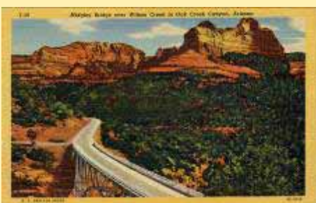
Y-39 Midgley Bridge Over Wilson Creek
