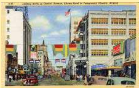
P-42 Looking North On Central Avenue,
