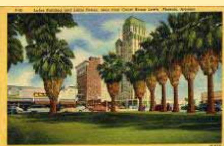
P-42 Luhrs Building And Luhrs Tower
