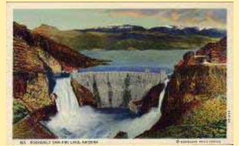
612 6A-H1501 Roosevelt Dam And
