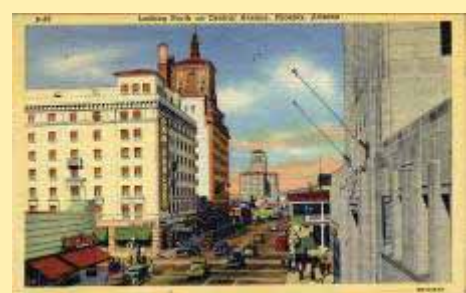
P-29 Looking North On Central Avenue
