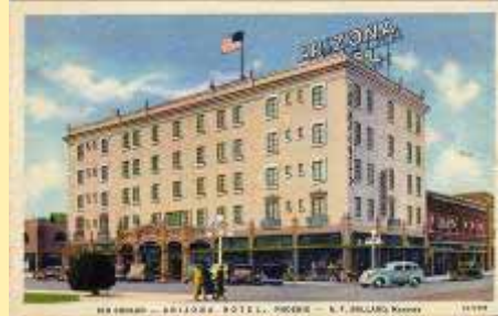
6A-H999 Air Cooled—Arizona Hotel, Ph
