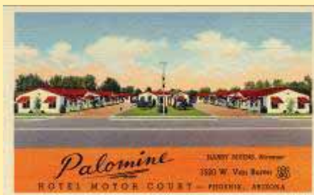
OB-H216 Palomine Hotel Motor Court
