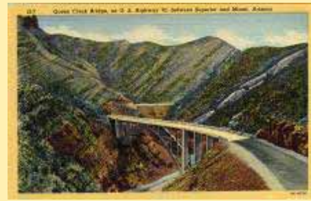
G-7 Queen Creek Bridge, On U.S. Highway
