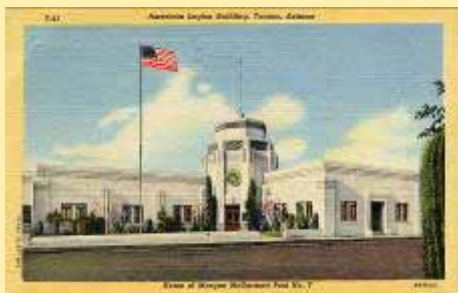
T-41 American Legion Building, Tucson
