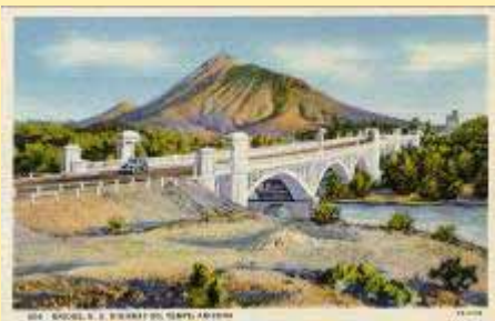
606 Bridge, U.S. Highway 80, Tempe, A
