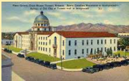
311 Pima County Court House, Tucson,
