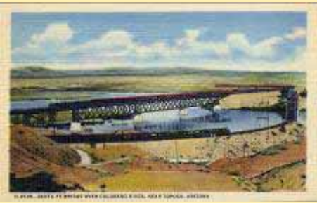
H-4509 Santa Fe Bridge Over Colorado R
