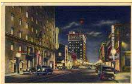
651 Looking South On Stone Avenue, Sh
